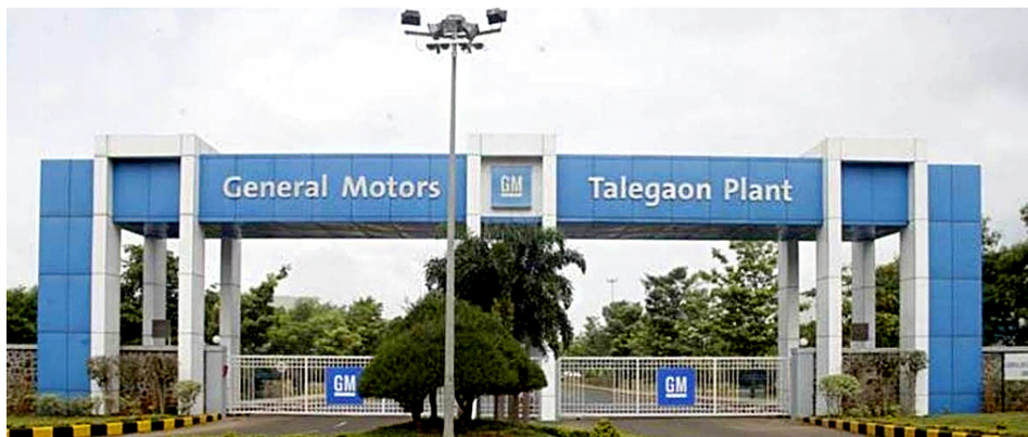
The main entrance of General Motors India’s Talegaon plant. (Chandrakanth Alsundkar)
